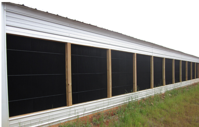
C. Tunnel inlet light trap.
