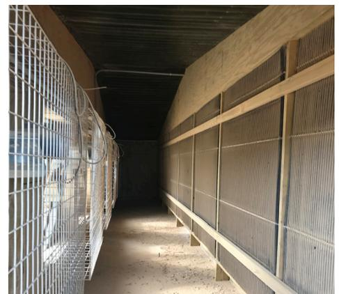
**D.** Light trap in a false wall in front of tunnel fans.
