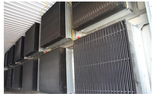
**B.** Light traps mounted over fans can reduce fan performance, and are not the best option in high-speed tunnel houses.
