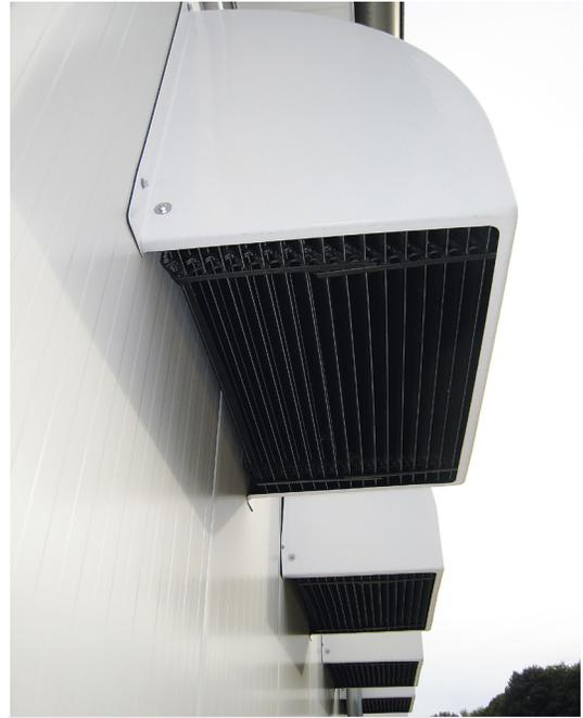
**F.** A perimeter inlet light traps installed in a box or wind proof cover.
