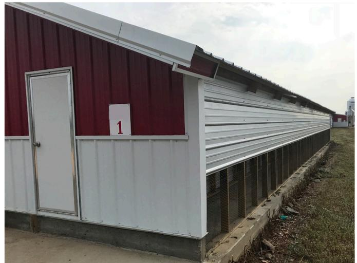
*When using evaporative pads, a shaded inlet area (similar to the images shown above) can eliminate the need for inlet light traps. Alternatively, the best option would be to use a light trap with a considerably lower light reduction factor and pressure drop.*
